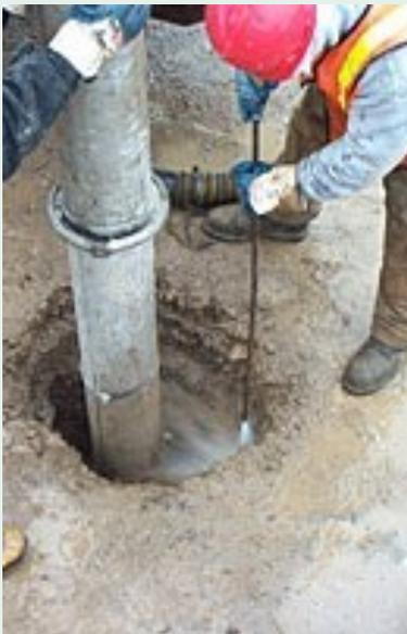
Hydro Excavation uses pressurized water to remove or move soil. The vacuum is used to transfer the soil to a debris tank. This allows a more safe way to excavate soil to locate underground utilities.
